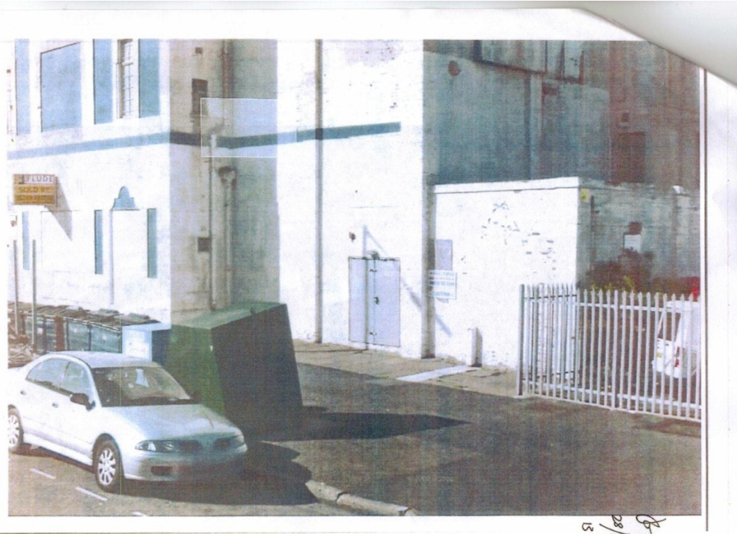
Photo 04: Past Use (2003 to Feb 2012) (source Mr J Escott Exhibit)
