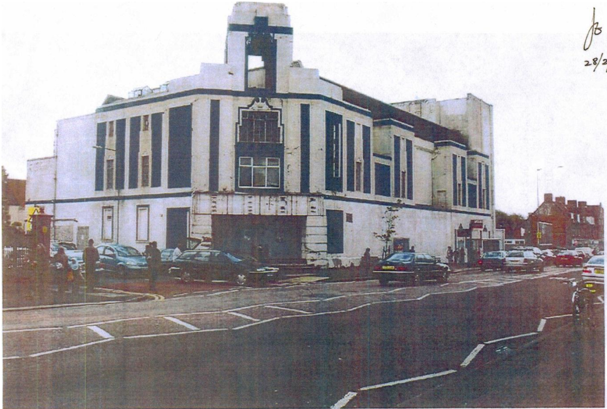
Photo 01: Past Use (2003 to Feb 2012) (source : Mr J Escott Exhibit)
